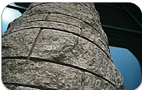
The entire building is covered in Tyndall stone from Flin Flon, Manitoba. This stone is 190 million years old, and, if you look closely, you can find fossils in it.
