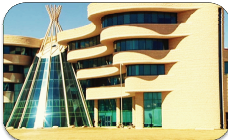
Each level of the building juts out further than the last. This maximizes sun in the winter and shade in the summer, saving energy.
